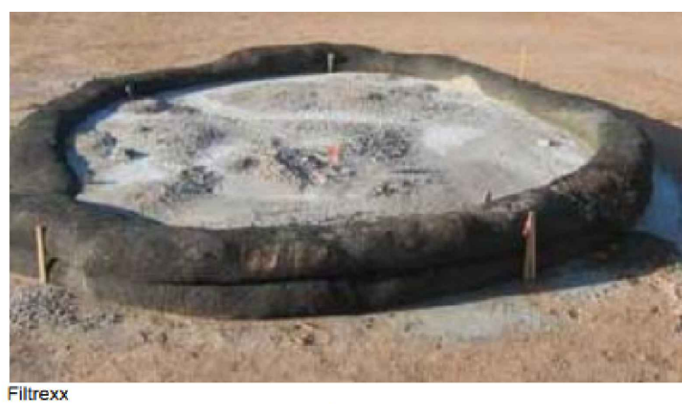
FIGURE 3.18 Typical Compost Sock Washout Installation
